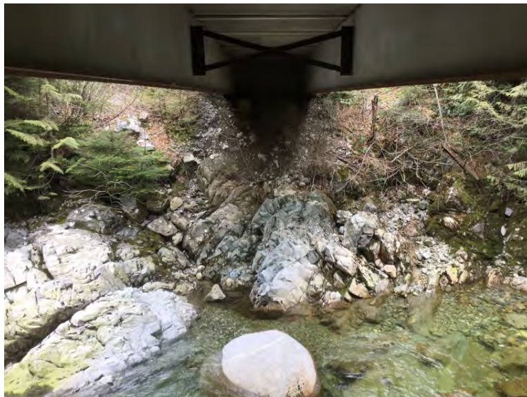
Left Bank Abutment when facing downstream
