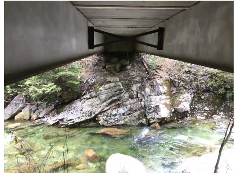
Right Bank Abutment when facing downstream
